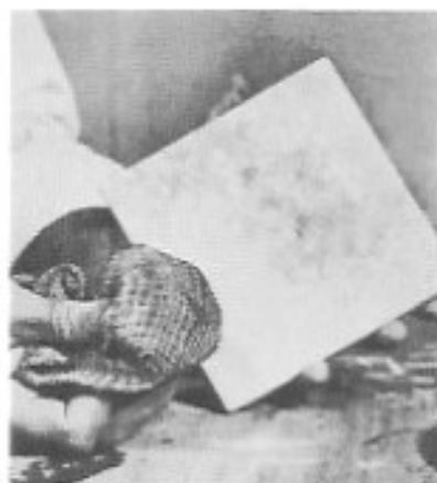
Cloth Printing: Rolling, printing technique; sponge inside for resiliency.
